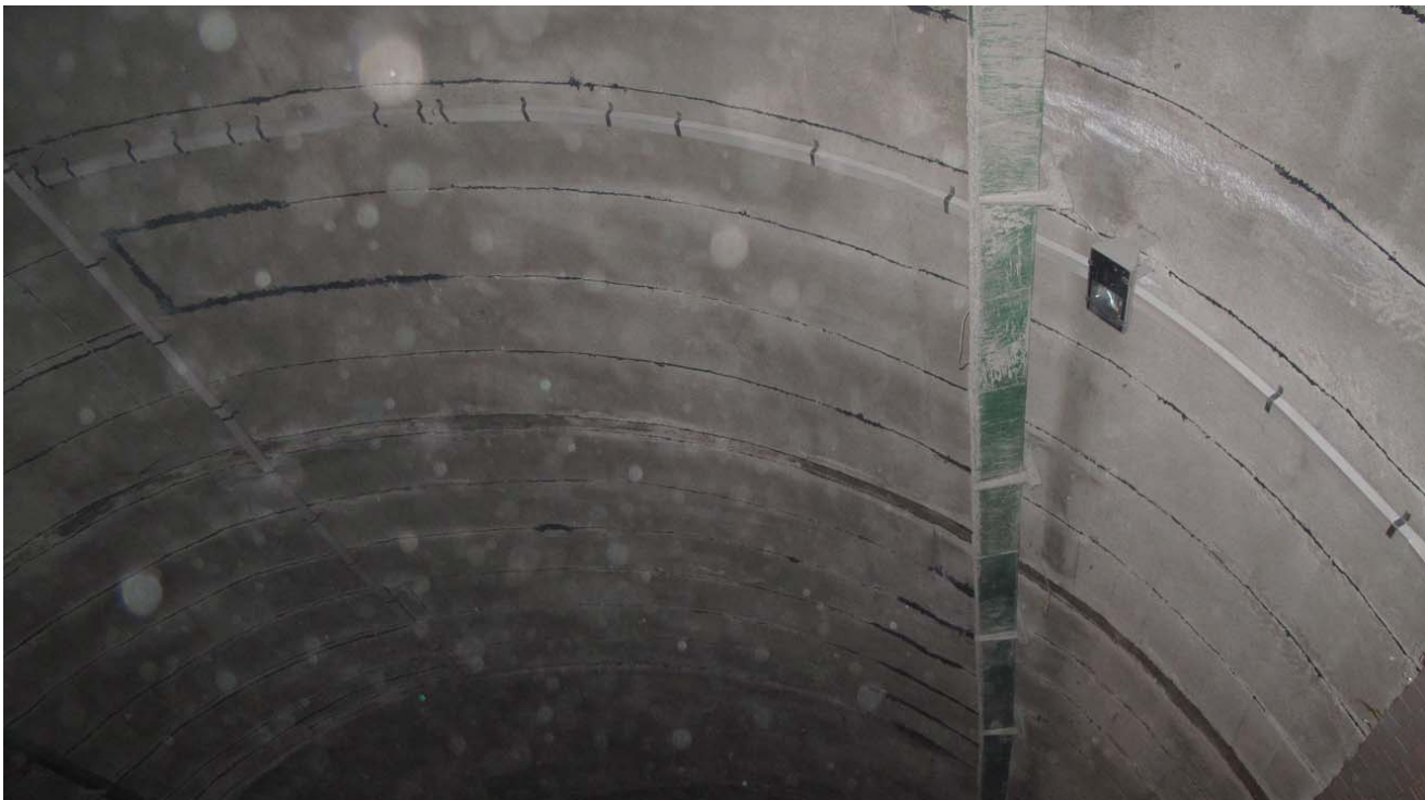
Installation of PVC trunking system
