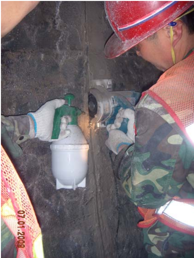
Saw Cutting Works – Lower Tunnel Lining
