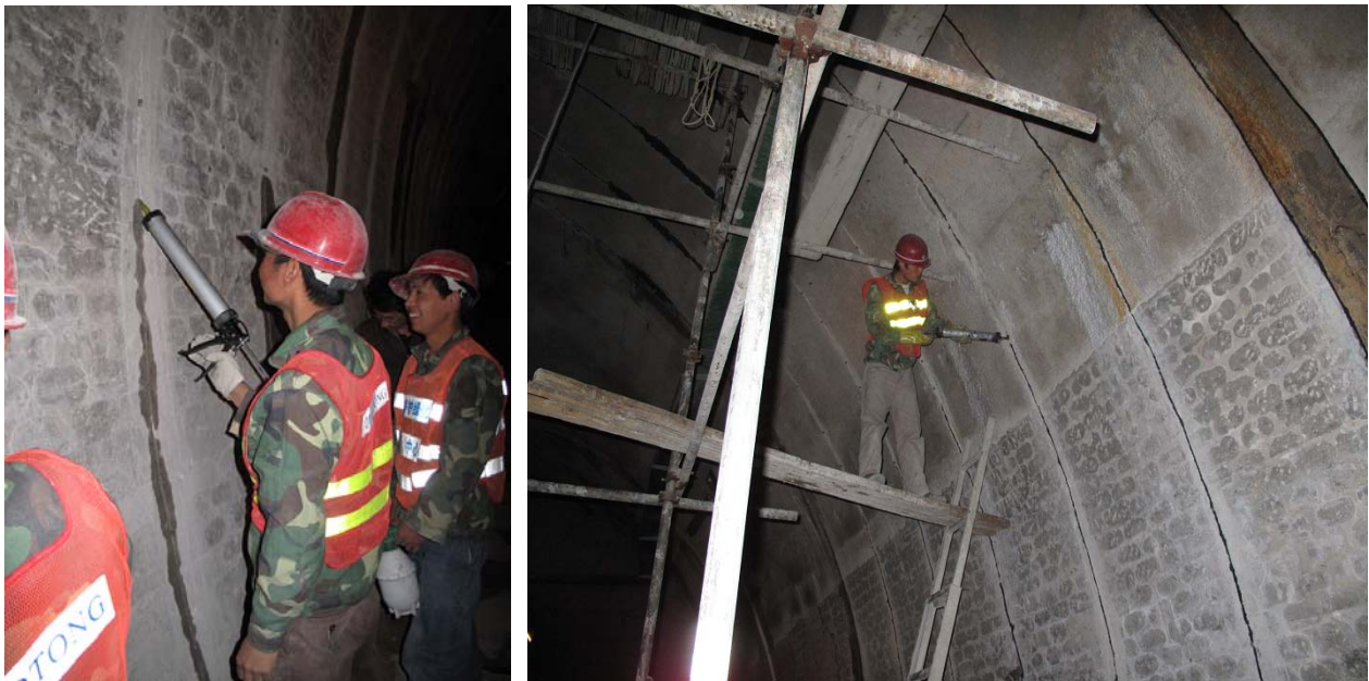
Grouting works at lower and upper level of the tunnel lining
