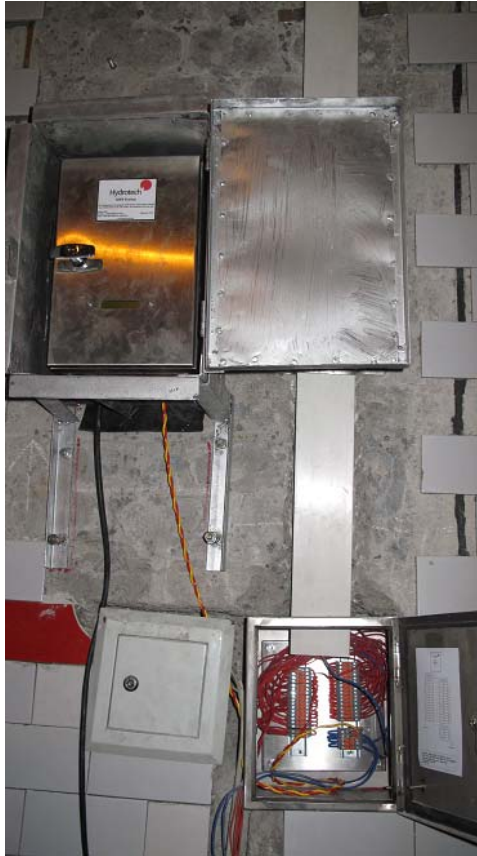
Control Unit to Junction Box Wiring Connection
