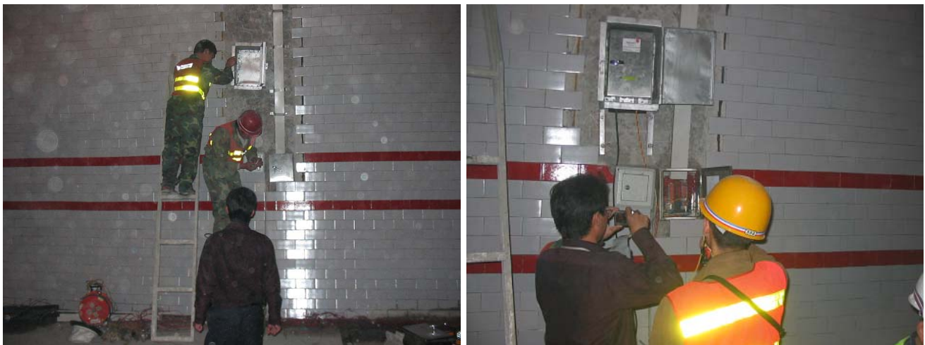
Installation of Junction Box and MPS Control Unit
