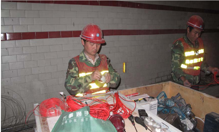
Preparation of feeder wires and installation
