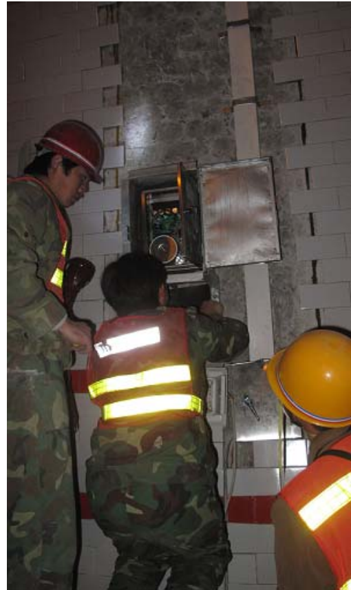
Control Unit to Junction Box Wiring Connection
