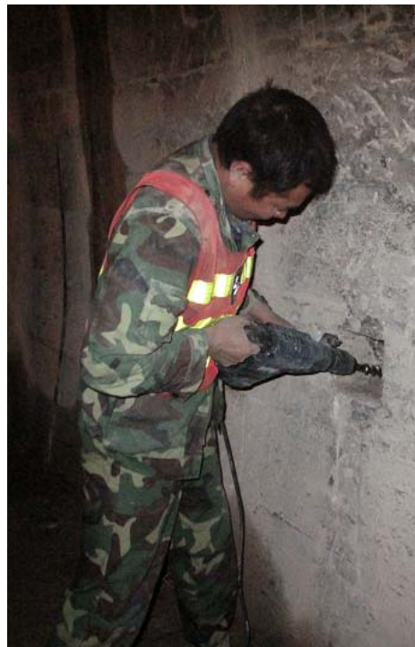
Cathode Installation
