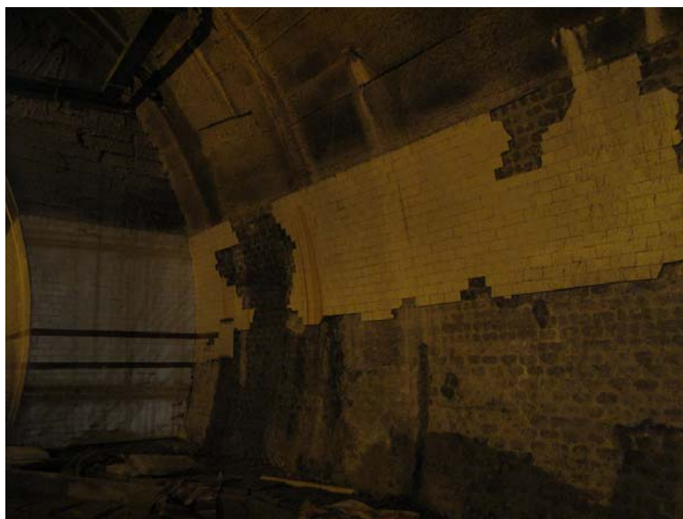
Signs of dilapidation of tiles and efflorescence
