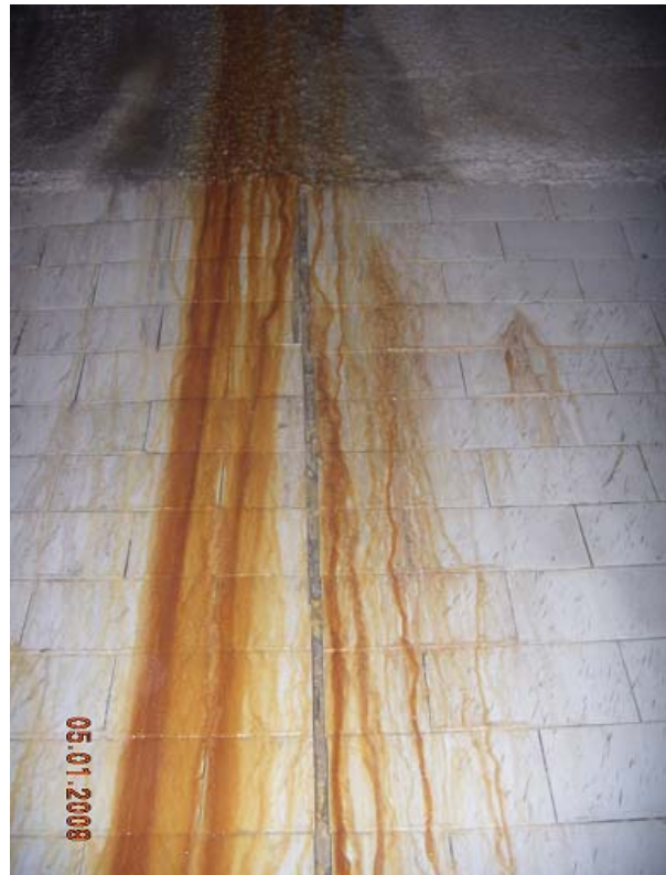
Signs of concrete degradation and failure of sheet membrane
