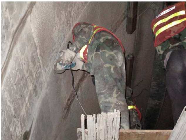
Saw Cutting Works – Upper Tunnel Lining
