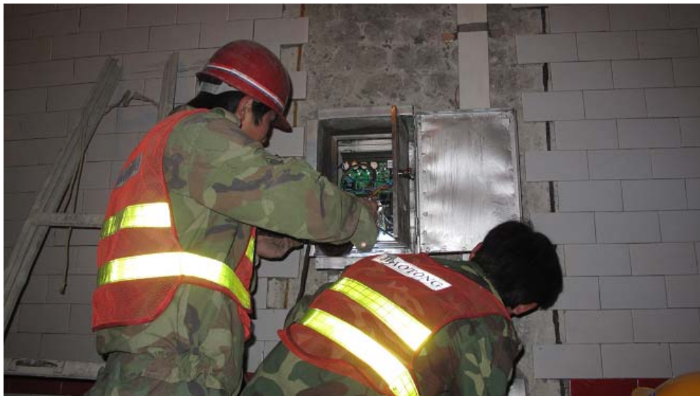
MPS Control Unit Installation
