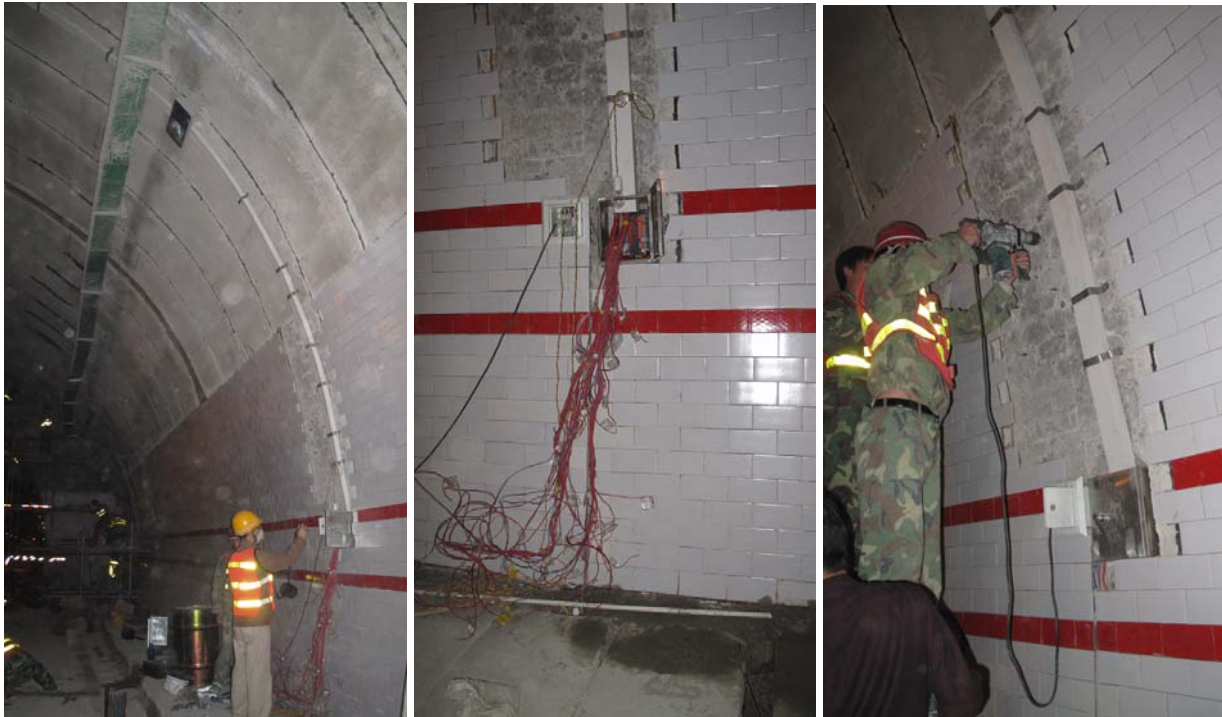
Connecting the feeder wires to the junction box
