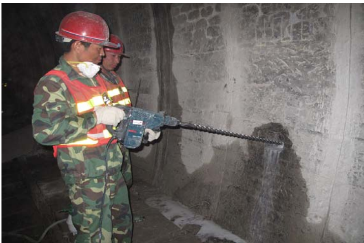
Checking of grooved depth and cleaning of grooves
