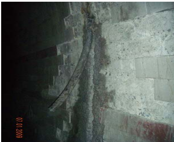
Existing Site Condition – Existing drain pipes was clogged, tiles are in dilapidated condition
