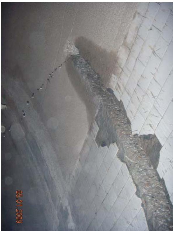
Signs of high water pressure behind the tunnel lining
