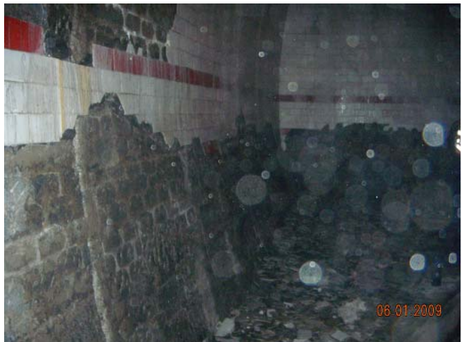
Existing Site Condition – Existing drain pipes was clogged, tiles are in dilapidated condition
