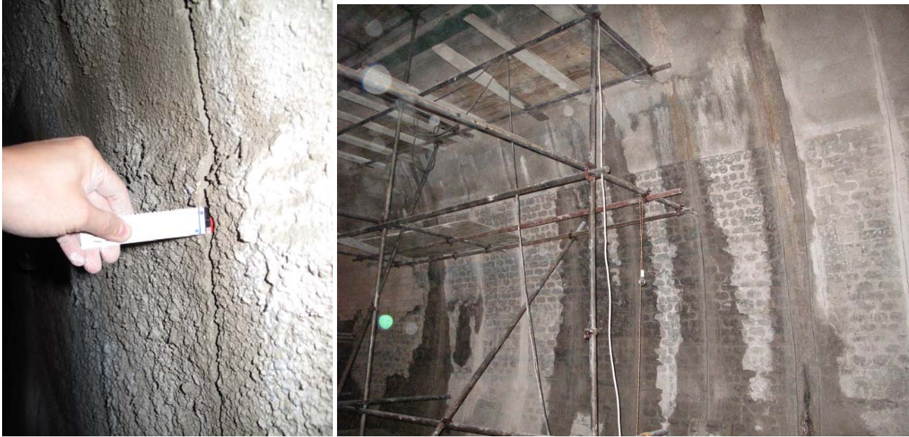
Checking of grooved depth and cleaning of grooves
