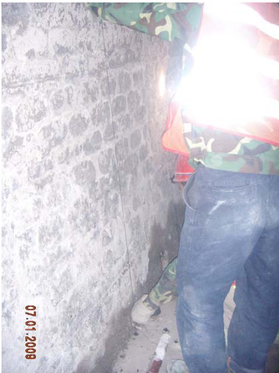
Setting-out of anodes, 100mm distance from the construction joints
