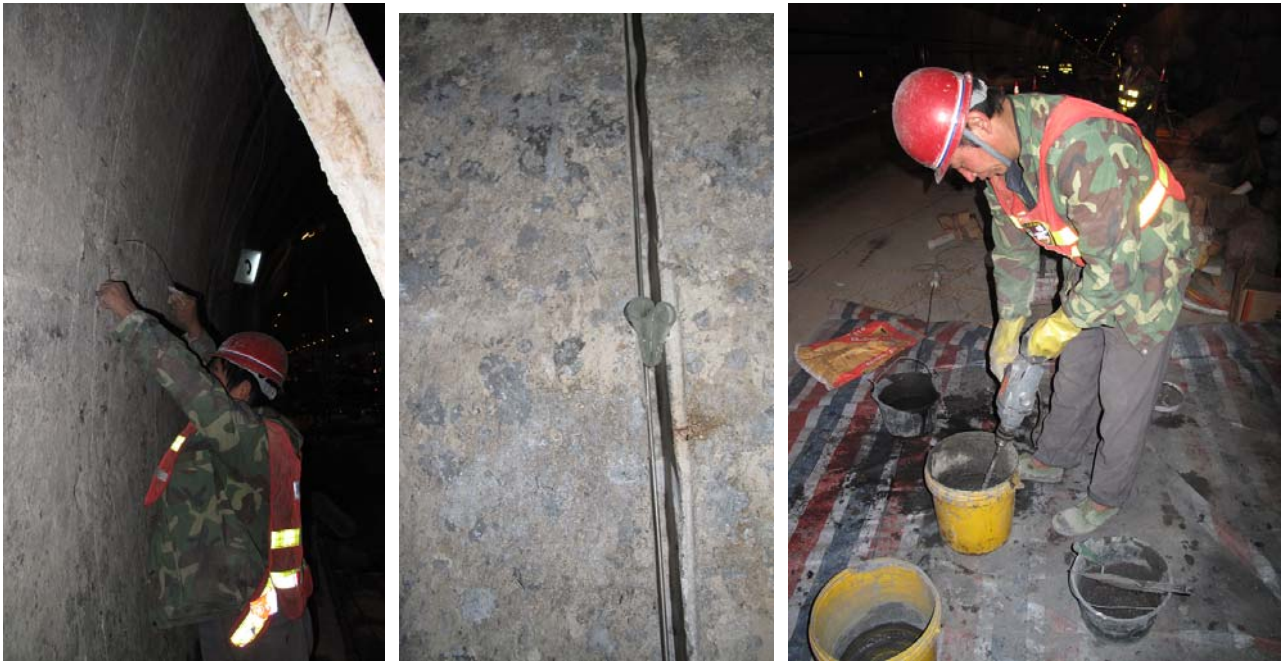
Titanium Wire Installation and grout preparation
