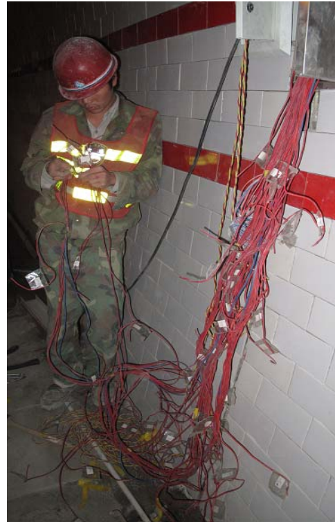
Feeder Wire Connection
