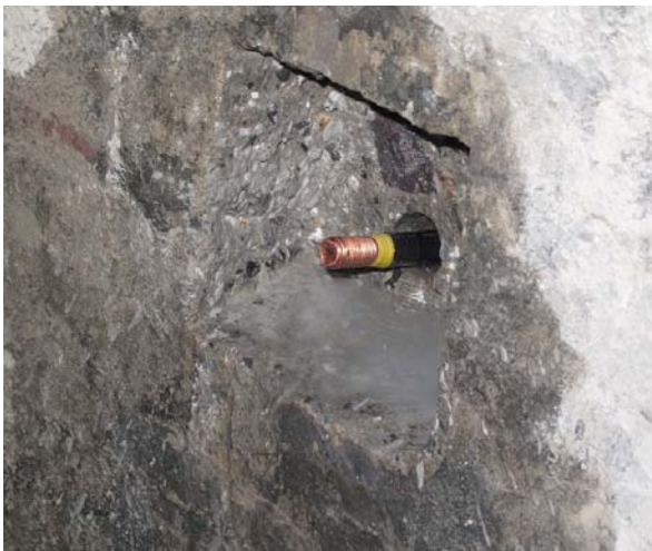
Cathode drilling and installation
