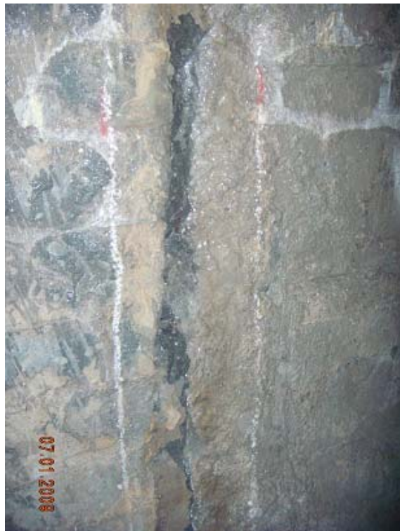
Setting-out of anodes, 100mm distance from the construction joints
