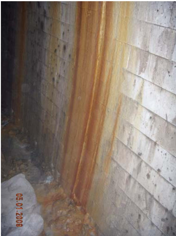
Signs of concrete degradation and failure of sheet membrane
