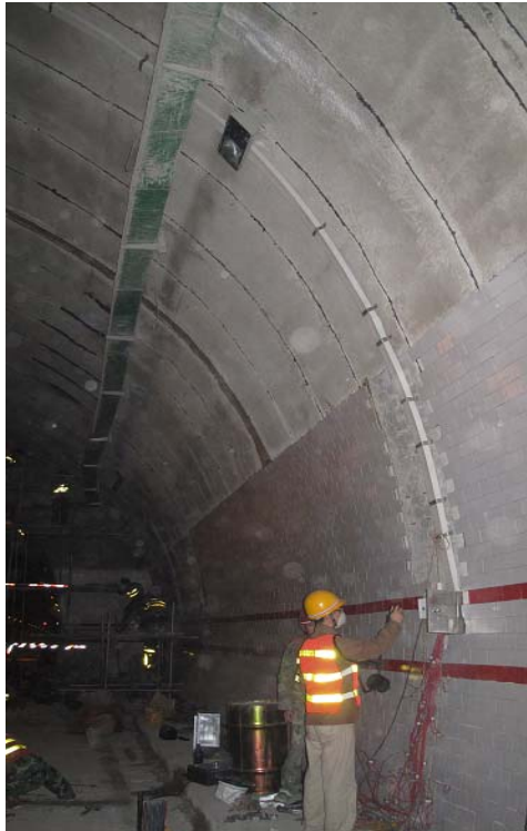
Trunking System Installation
